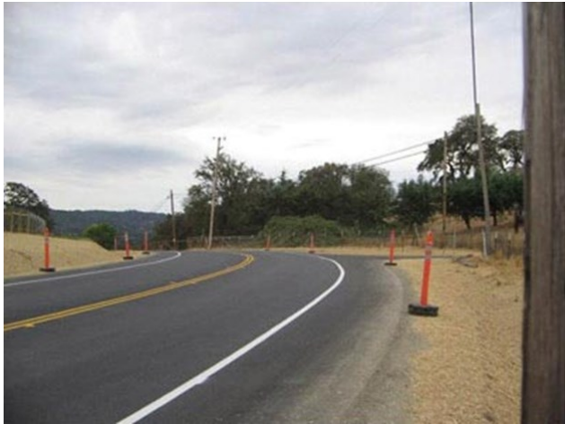
This photo shows McCourtney Road after the safety improvement project with temporary pylons still along the shoulder. The project widened the roadway and leveled off the shoulder.
