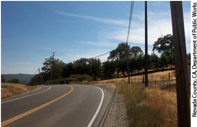
Shown here is McCourtney Road in Nevada County, CA, before the implementation of a safety project to improve the highway's sharp curve to the left.
